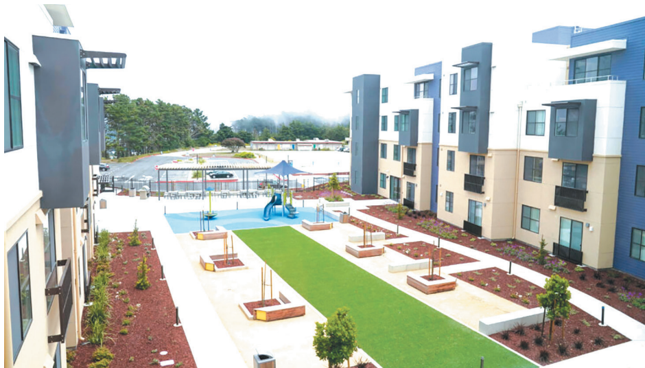
HOUSING COMPLEX for teachers and education staff of Jefferson Union High School District in Daly City. A. Vásquez/AP Photo
