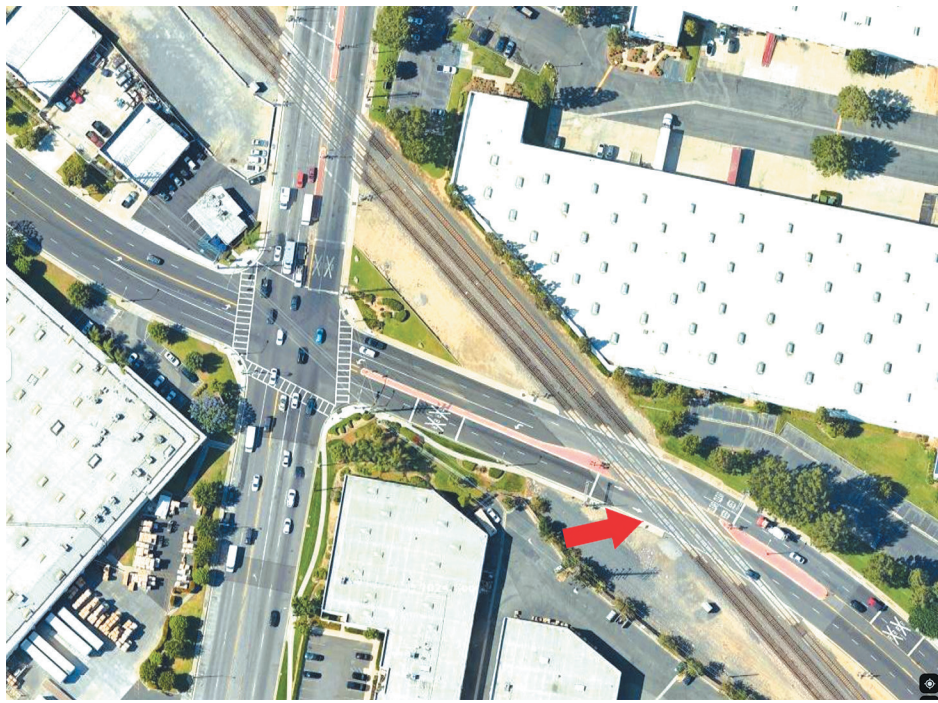
CURRENT CROSSING: The Norwalk Boulevard and Los Nietos Road crossing (arrow). Nearly five trains per hour (109) cross daily; 50 of those are passenger railroad cars, while 59 are freight. The grade separation will improve safety, reduce emissions, enhance mobility and connectivity, and promote economic equity while improving efficiency for rail traffic.
